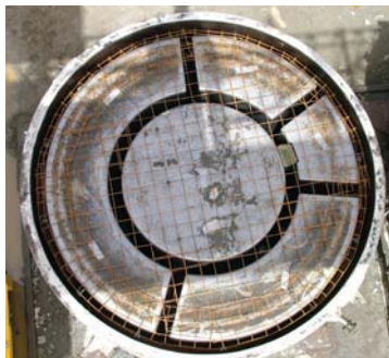
Inverted Mould with Reinforcing Ready for Concrete
